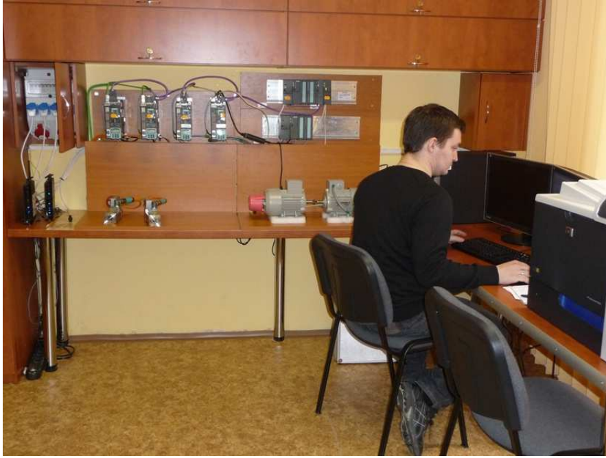
Laboratory for application of industrial control systems
